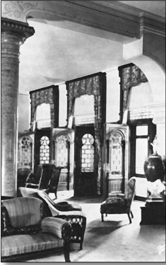
The Rotunda Room used as the main lobby.
