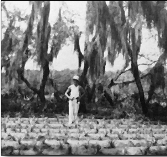
Pineapples that eventually were dug and cleared with a grubbing hoe.
